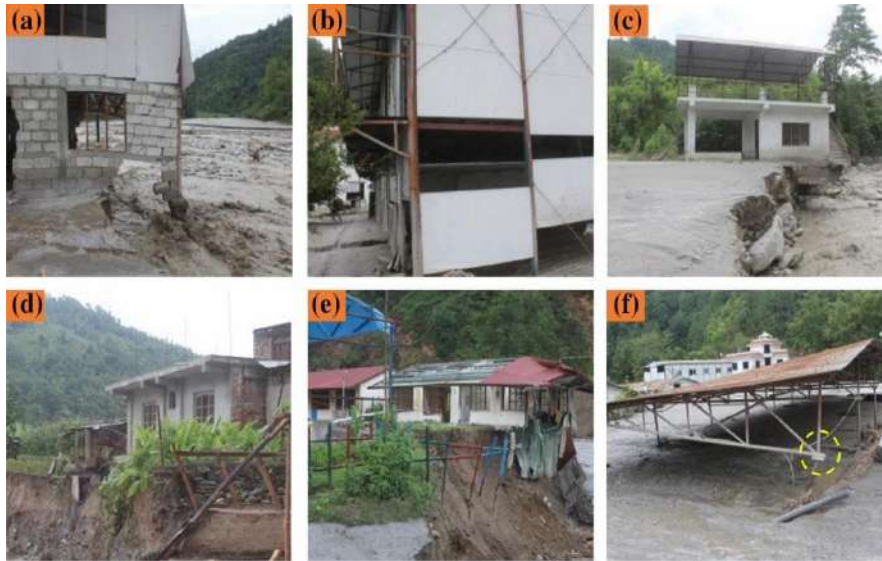
Figure 2. Landslide contributing to flooding hazard.
