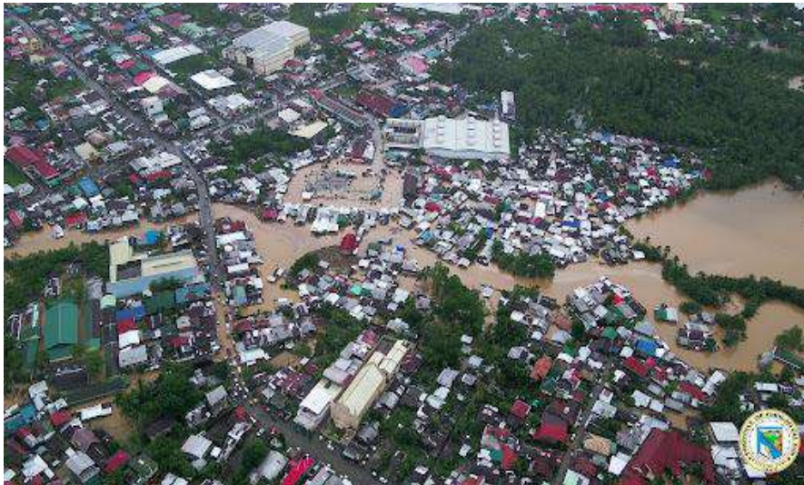
Figure 4. Poor water drainage network
